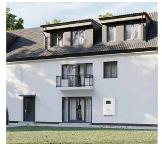
Residential Project in the United State 6kW
