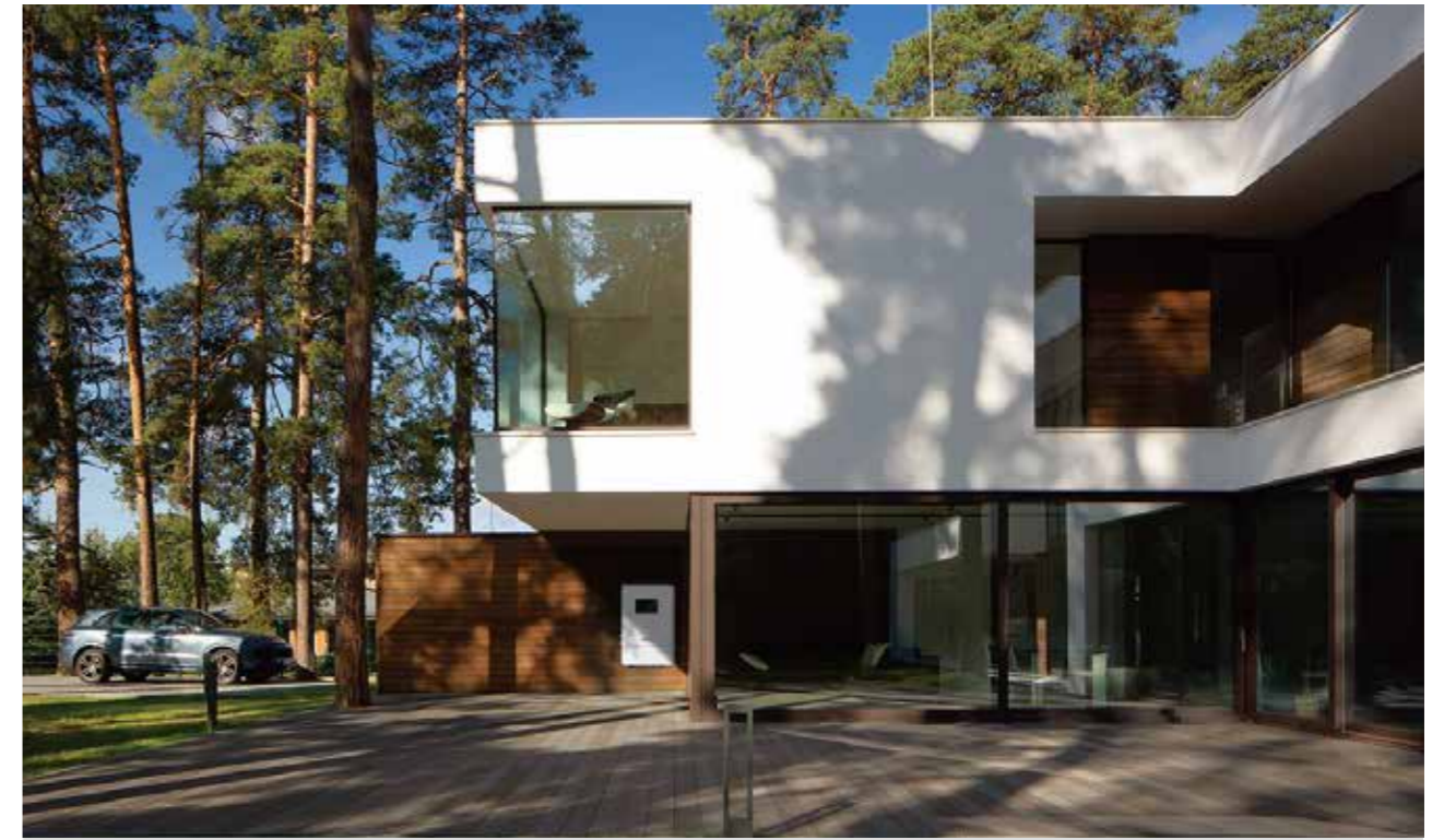
Residential Project in the United State 10kW
